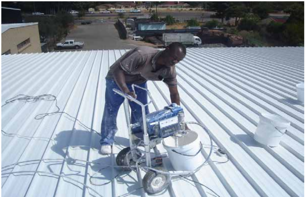
Picture.1. AGNA coating a metallic roof with Ceratech
