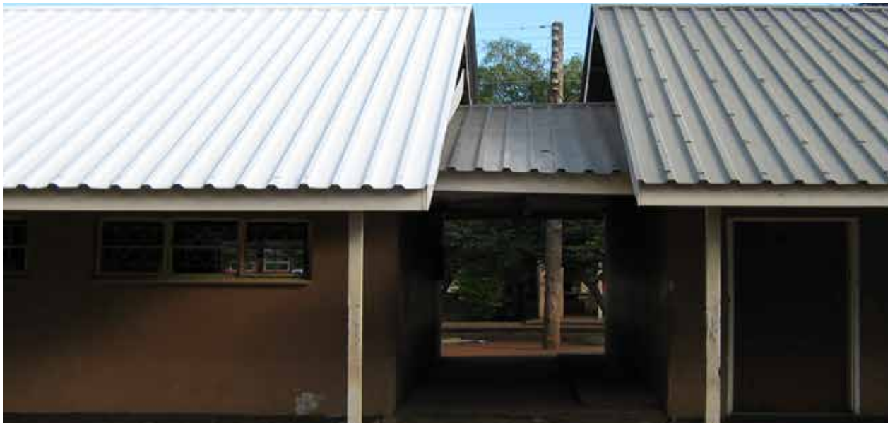
Picture 2. Ceramic Painted (white) and unpainted metal roofs (dark) of semi-detached buildings at Ramotswa CJSS.
